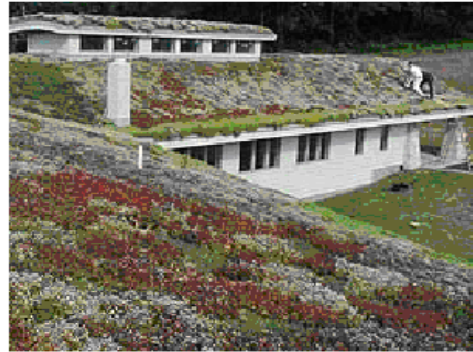
Building with Green Roof
